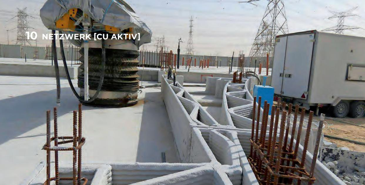
Building, framework and reinforcement – in Dubai start-up Apis Cor built a 3D-printed office building
