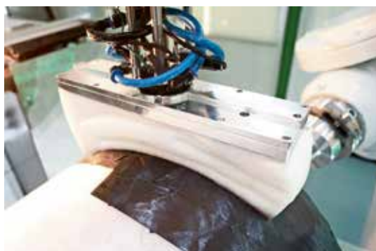
Placement of local dome reinforcement patches with FPP
