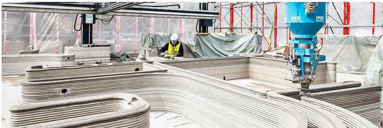
Fig.29-1: Particle-bed technique (up left), Mortar strand depositing technique (up, right); (below) Peri GmbH, building a two-story house in Beckum, 2021
